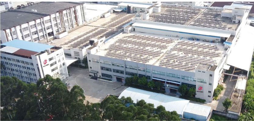
Amitime Manufacturing Center in Zhongshan, Guangdong
